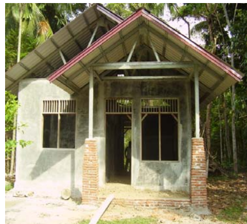
Figure 46. LGS structure for houses
