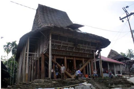
Figure 47. Building Stock is still exist due to bracing
