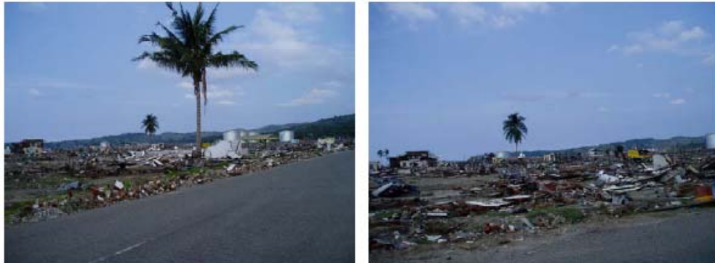
Figure 34. Pertamina Oil Depot, Krueng Raya
