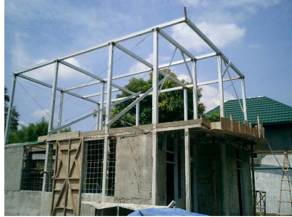
LGS (Light Gauge Steel) structure
