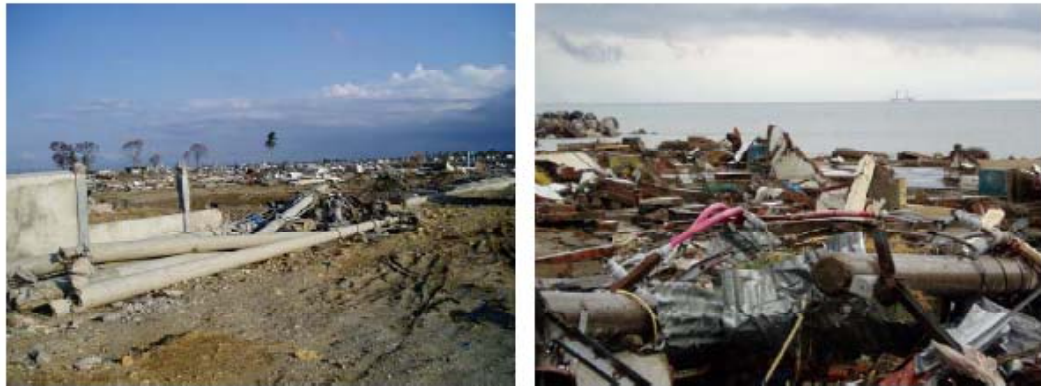
Figure 30. Main Power generating plant in Banda Aceh
